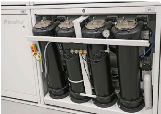
MicroPur® modules are equipped with four filter housings, each containing two filter cartridges. The cleaning capacity per module is 400 l/min.
