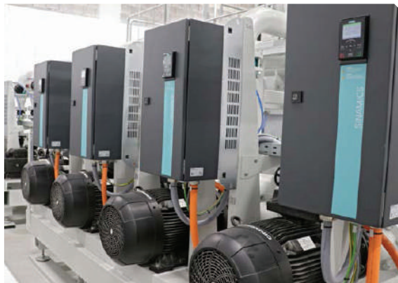
The five KNOLL process pumps for the aqueous solution system can be seen in the foreground. They pump the cleaned medium back to the machines as required. In the background are the three somewhat smaller filter pumps, all of which are frequency-controlled.
