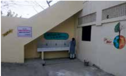
Renovated hand wash area
