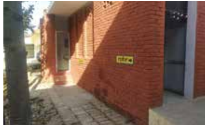
Cleaned and repainted washrooms
