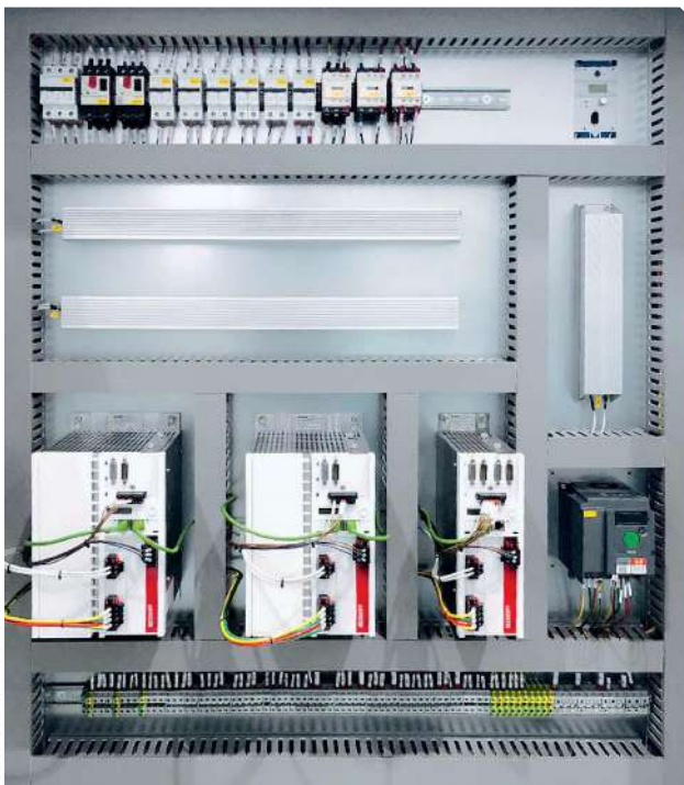
AX5000 Servo Drive from Beckhoff in the laser cutting machine control cabinet
